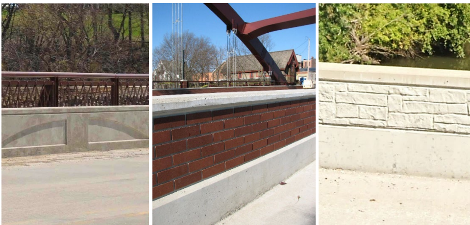
Figure 5.8.1.2.5-4. Examples of Barrier Traffic Face Treatments
